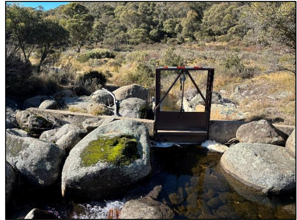
Plate 6. Upstream weir sluice gate at entrance to snowmaking ponds (east)
